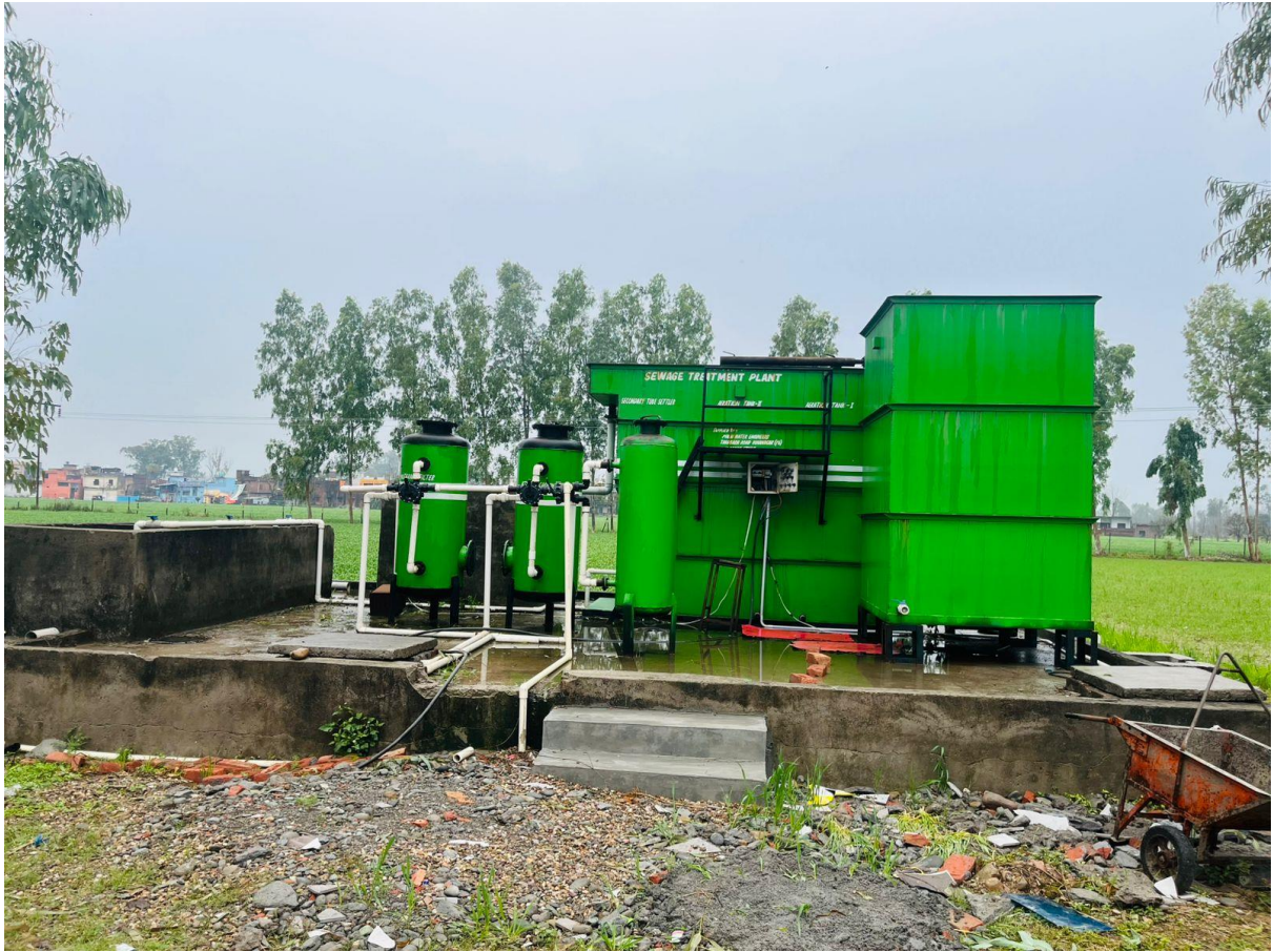
Sewage Treatment Plant
